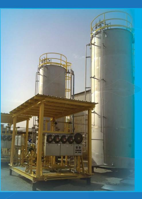
TANK store the chemicals which need to be injected into the process or systems. The tanks usually are either of horizontal cylindrical having dished end or vertical cylindrical with flat/conical/ dished bottom and flat/dished top or of rectangular construction. The applicable design codes can be as per the ASME Sec VIII U-stamped, API 650, UL 142, BS 2654, BS 4994. The material of construction can be CS, SS304, SS316, SS316L or GRP. Tanks can be coated as per the client's requirement.
